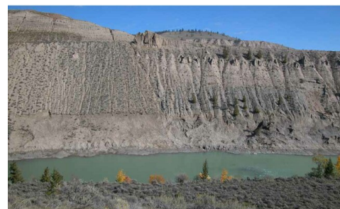
Figure 5.10: Rill and gully erosion along the Chilcotin River [GSP*10].
